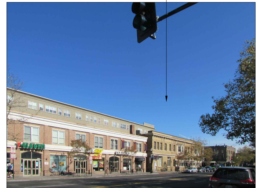
③ U STREET (LOOKING EAST)
